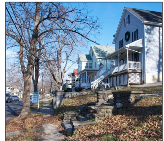
Above (top to bottom): Residential street with sidewalk system in good condition; ADA compliant ramp at corner of NYS Route 52 and Elm Street; and view of bluestone sidewalks, which need to be re reset, repaired or replace due to tree uprooting sidewalk segments.
