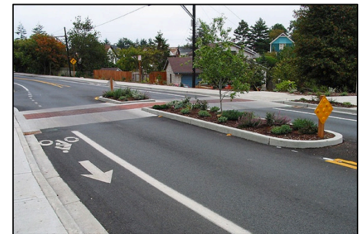
Above (top to bottom): Illustration showing mini round about, which could be utilized to calm traffic entering the Village from arterials; image showing textured surface crosswalk to alert drivers when they are approaching a pedestrian crossing and view of a midblock median island with textured surface crosswalk to provide safe crossing for pedestrians. These types of traffic calming measures are recommended for the Village of Walden.
